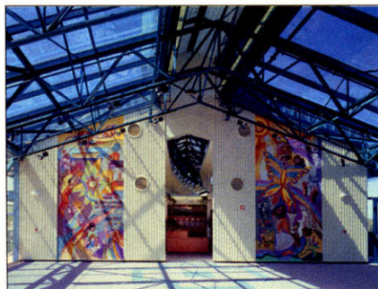
Gable manufactured joists support glass panels and clerestory.
