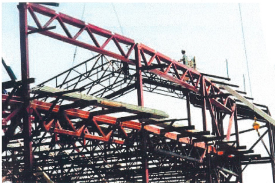
Tube steel girder trusses span along circumference of the building, with joist top chords extending to form exterior walkways.
