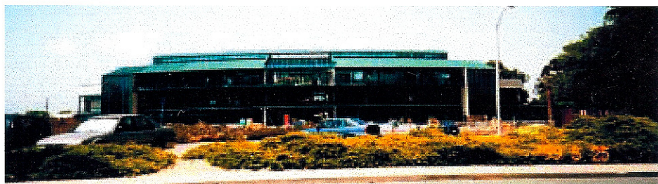
Front view of Pittsburgh Civic Center.
