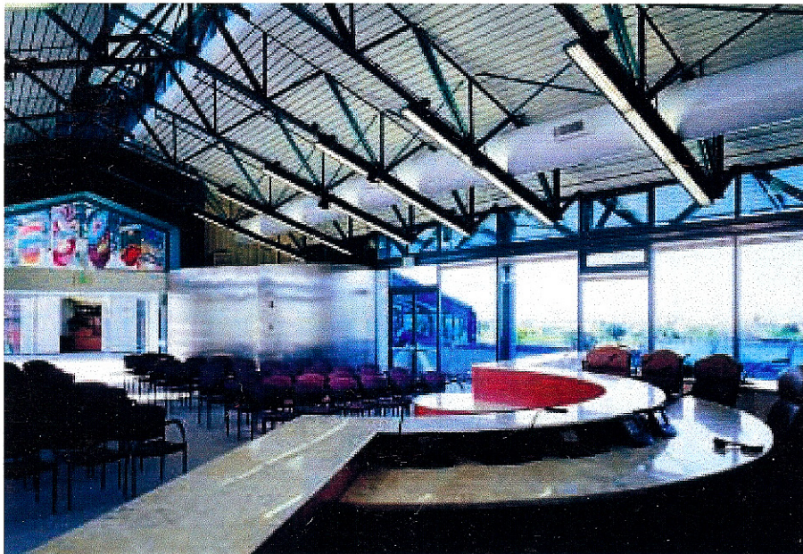
Exposed steel joists and girders are on display at the 3 rd floor council chamber.
